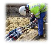
The cable joints are used to connect low, medium or high voltage cables. The type of cable joint sizes, shapes and configurations vary according to the voltage, structure, insulation and the number of cores of the cable to be jointed. The joints provide electrical insulation as well as mechanical protection and strength. The electrical connection is made in various ways and can crimping, or use of mechanical connectors, soldering, etc.
